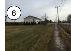
6 CONSTRAINT Home is located in close proximity to existing right-of-way limit.
