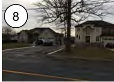
8 CONSTRAINT Homes are located in close proximity to existing right-of-way limit
