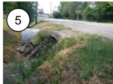
5 OPPORTUNITY Improved drainage through provision of a single, properly sized culvert. Low impact development to be employed.
