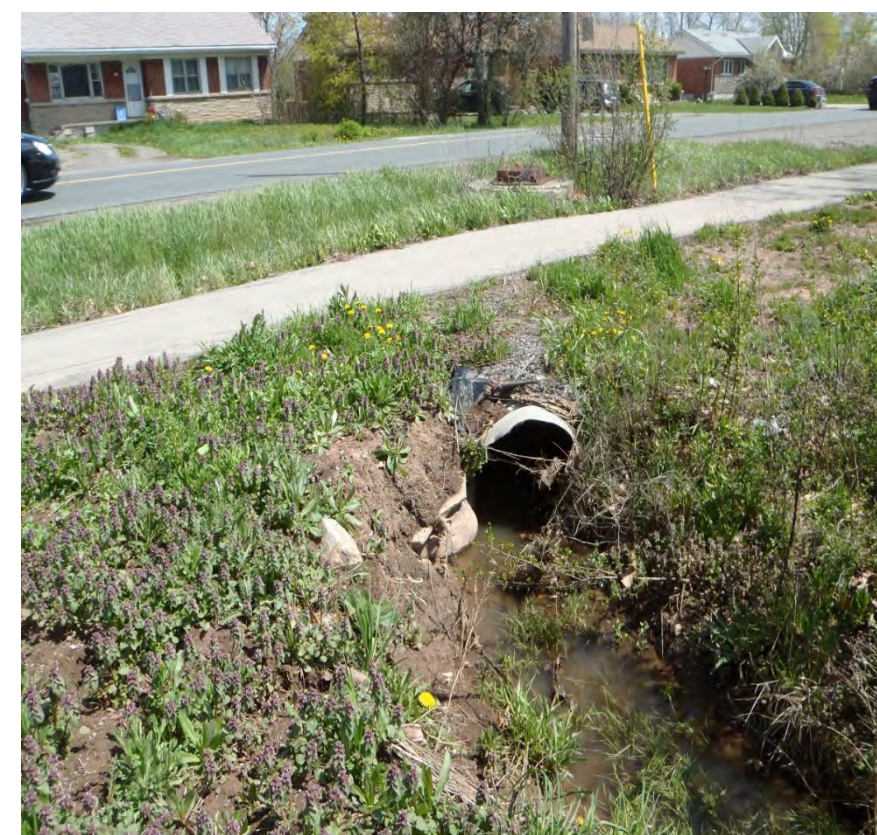
Watercourse Crossing 5.2-Upstream
