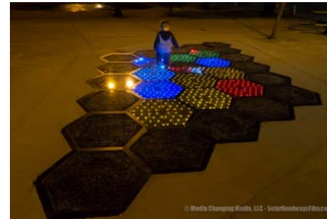
Solar-powered pavers at installation in Sandpoint, Idaho. Collected energy can be stored to power street lights and/or the light the actual panels themselves.
