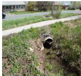
Watercourse Crossing 5.2-Upstream
