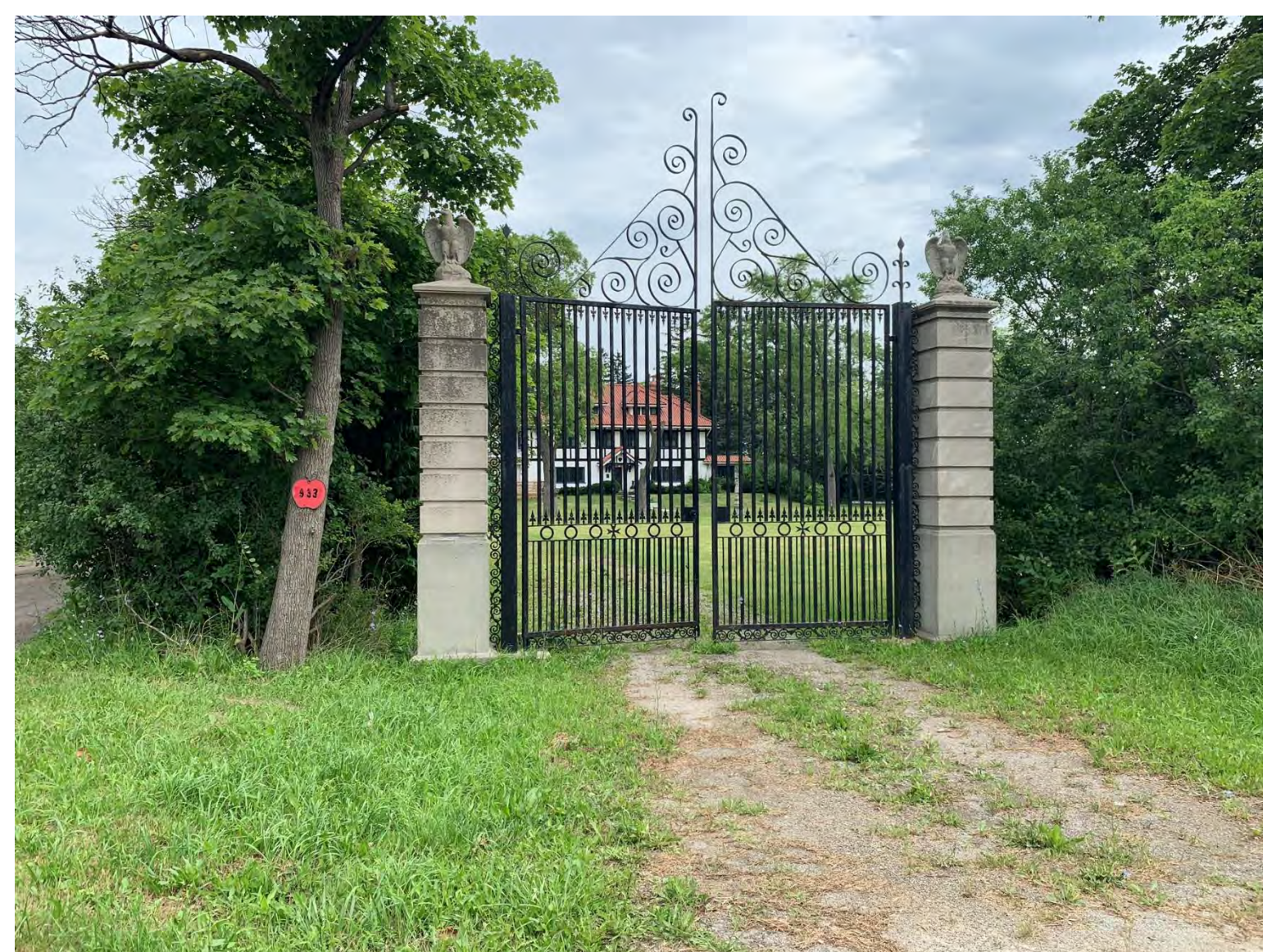
Narrowly setback gate at 929-933 Highway 8 (listed)
