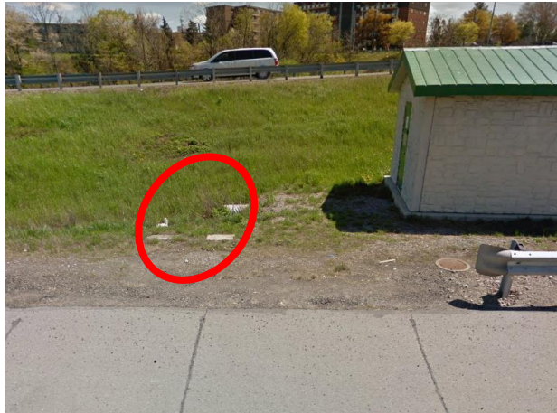
Figure 36: Culvert/Utilities North of HCS07B
