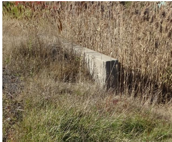
Figure 27: Fixed Objects Protruding More than 100 mm Above Ground
