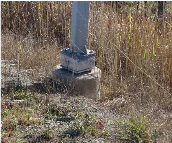
Figure 27: Fixed Objects Protruding More than 100 mm Above Ground
