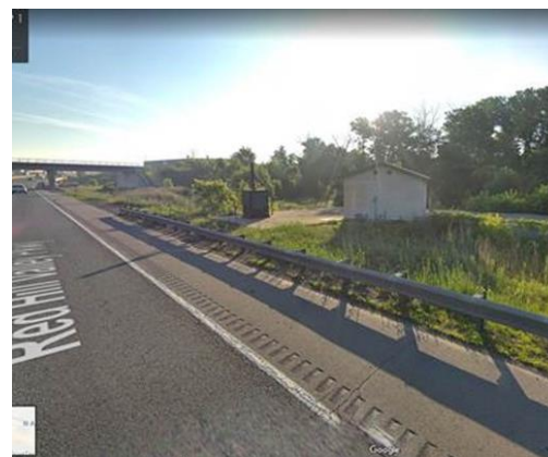
Figure 33: HCS07C near Barton Street
