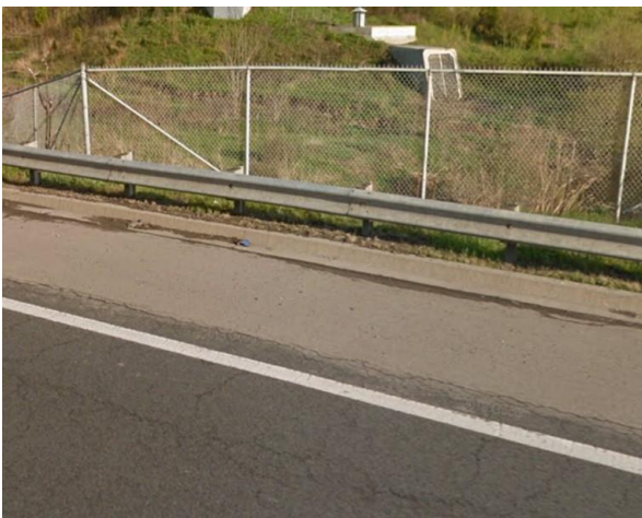
Figure 23: SBGR with Barrier Curb
