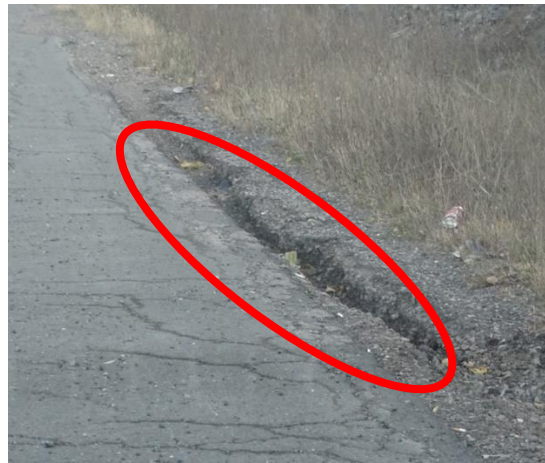
Figure 30: Shoulder Erosion
