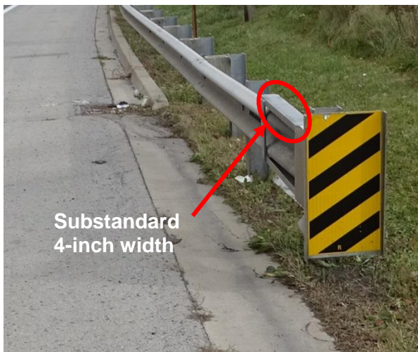
Figure 21: Substandard 4-inch Extruder
