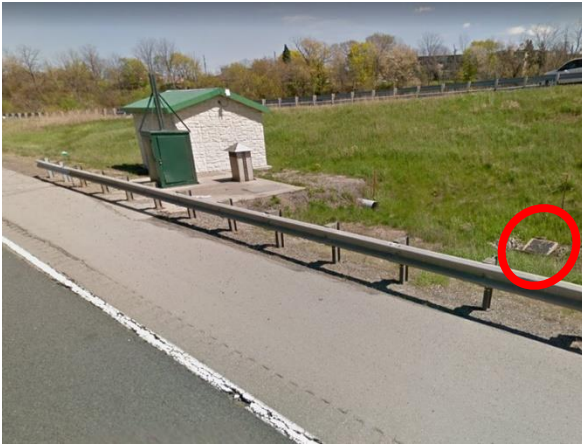
Figure 35: Catch Basin South of HCS07B
