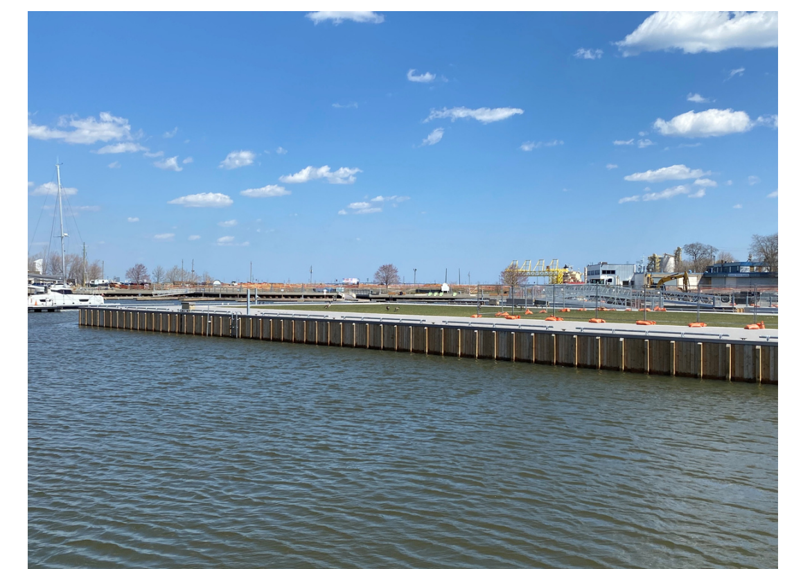
Piers 6 & 7 Shorewall Rehabilitation, Fish Habitat & Public Boardwalk
