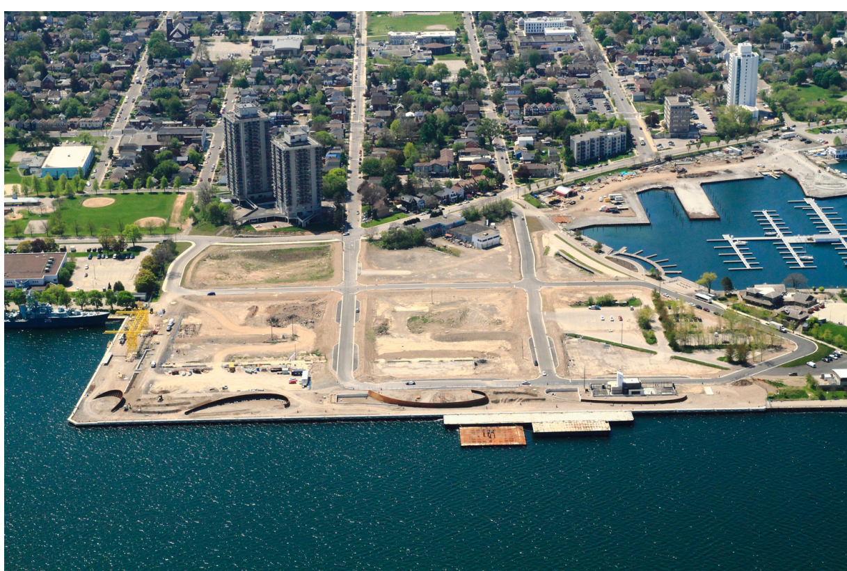
Pier 8 Servicing (Underground & Road) Infrastructure
