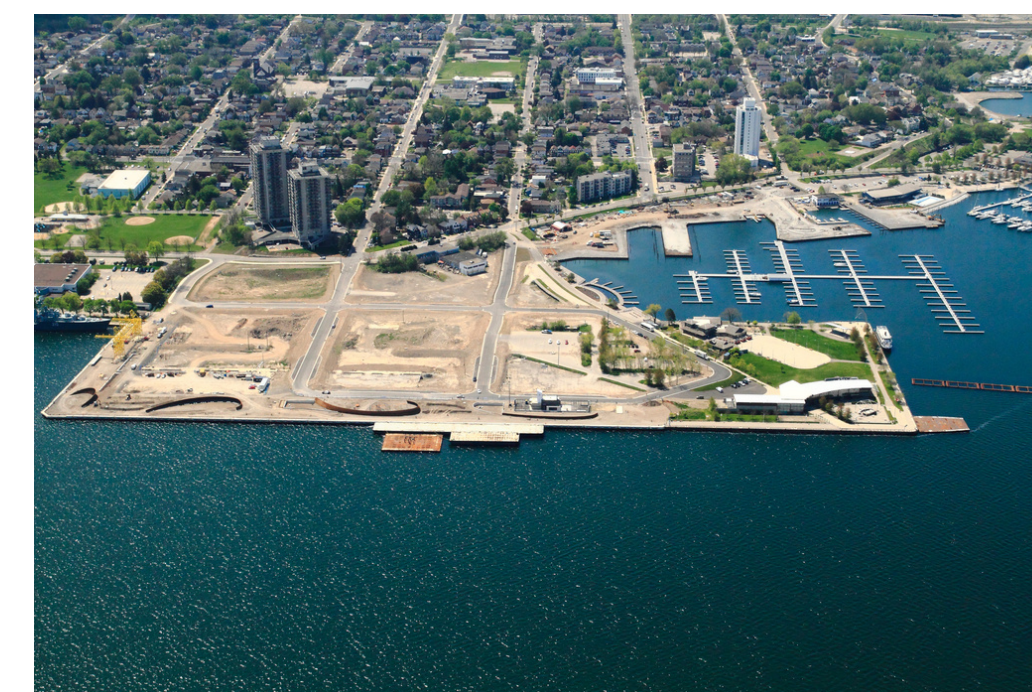
Pier 8 Shorewall Infrastructure Rehabilitation & Renewal
