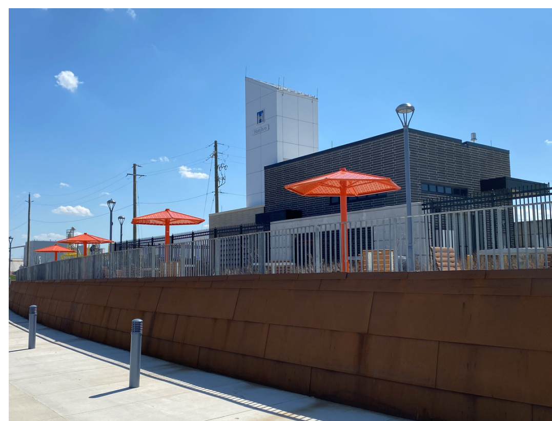
Pier 8 Sanitary Pumping Station Infrastructure
