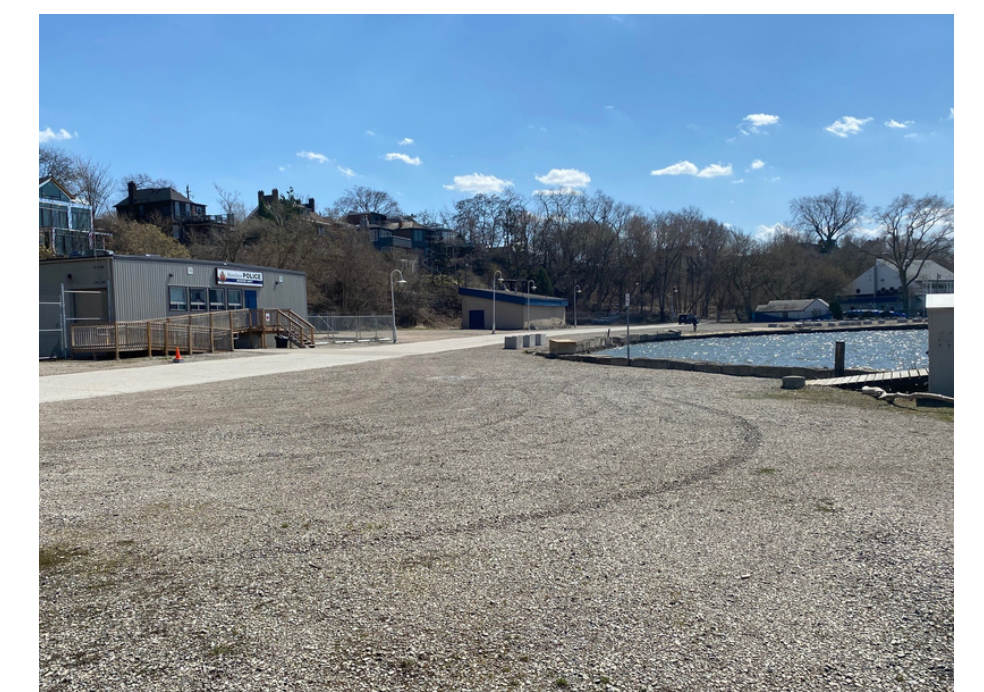
Pier 8 Shorewall Infrastructure Rehabilitation & Renewal
