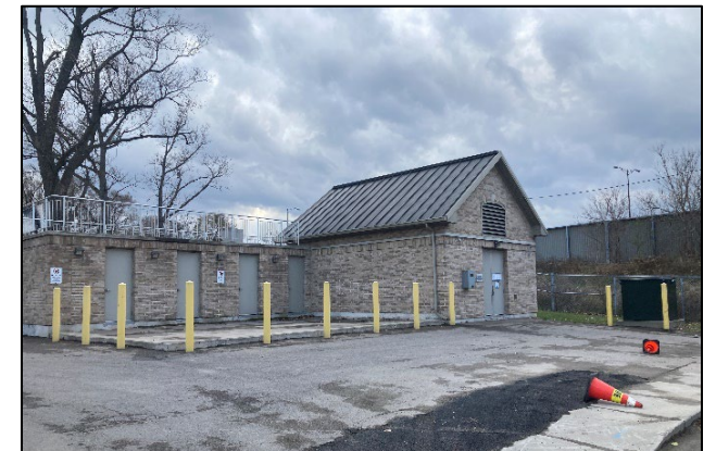
Existing Grafton Pumping Station
