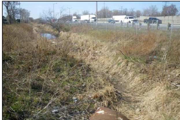
Existing Eastport Ditch
