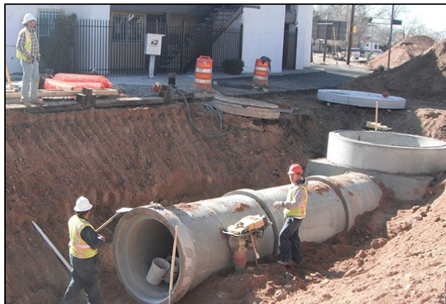
Storm Sewer Installation
