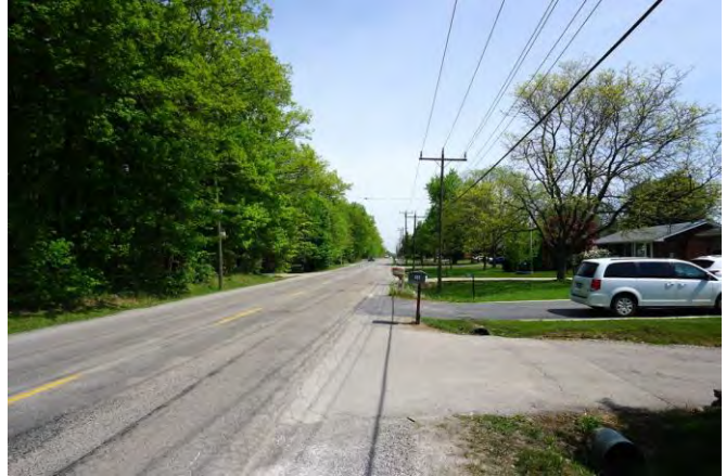
Photograph 4: View of Glancaster Road, looking north (AECOM, 2021)
